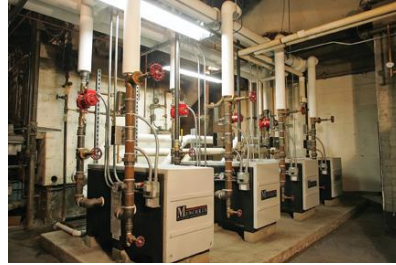
Left: A “typical” older, larger, less efficient boiler - Ashland, WI County Courthouse.
